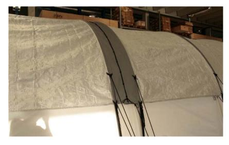
Place the flysheet with laces along/against the flysheet with eyelets. By connecting two flysheets it is important to start in the middle, and sew towards each side. The middle of the flysheet with eyelets is marked with a black line and the middle of the flysheet with loops there is two loops, one for each direction.
